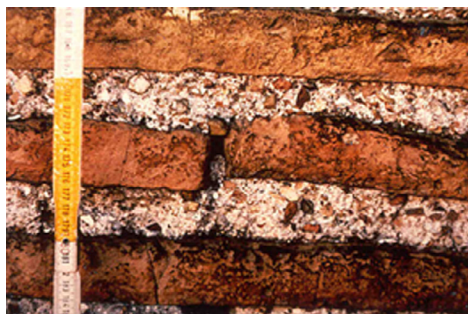
图4：意大利拉文纳圣维塔莱大教堂厚砂浆接缝 Figure 4. View of thick mortar joints of St. Vitale basilica in Ravenna (Italy)
