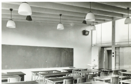
图3: 弗拉基米尔·卡尔菲克和约瑟夫·哈尔万奇克, 斯洛伐克布拉迪斯拉发实验学校, 1956-57年。双面采光教室内部, 玻璃墙板可与走廊建立视觉联系。 Figure 3. Vladimír Karfík and Jozef Harvančík, Experimental school, Bratislava, Slovakia, 1956-57. Interior of the bilaterally lit classroom with a glazed wall panel allowing a visual connection from the classroom to the hallway.
