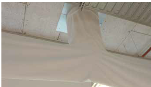
图 11: 送风管（织物）及排风管 Figure 11. Supply (fabric) and exhaust ducts
