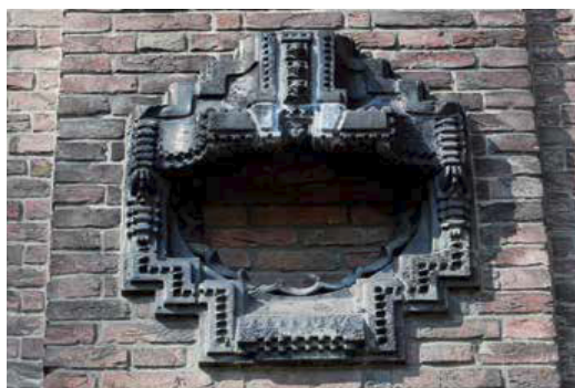
图 9: 狮头状通风口 (内部可见填充物) Figure 9. The lion head like ventilation openings (filling visible inside)
