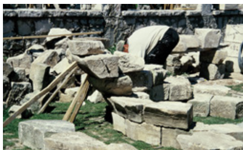
图 1: 回收散落的石块在地面拼装的宣礼塔阳台 Figure 1. Minaret balcony assembled on the ground with recovered blocks
