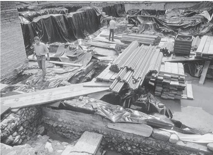
图 3：由于计划不周，挖掘过程中的典型糟糕情况。在等待建造临时庇护所的过程中，考古基址被聚乙烯薄膜覆盖。在此期间，雨水淹没了大部分挖掘区域，用于建造掩体的材料被直接放在了考古遗迹的上面。如果对活动的时间和顺序进行适当的现实规划，许多潜在的有害情况是可以避免的 Figure 3. Typical bad situation during excavation due to inadequate planning. Archaeological features have been covered with polyethylene sheeting while waiting for a temporary shelter to be constructed. In the meantime, rain has flooded much of the excavated area, and the materials to be used to construct the shelter have been placed directly on top of the archaeological features. Many potentially harmful situations can be avoided with proper realistic planning of the time and sequence of activities
